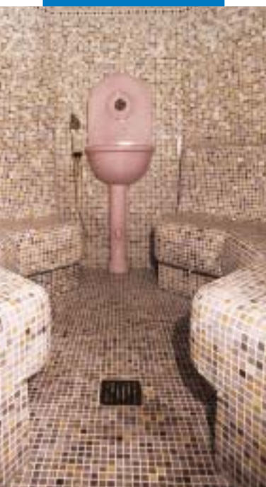
An example of an installation glass mosaics in a turkish bath - Park Hotel Gritti - Bardolino (Verona), Italy
