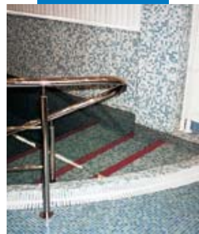
Laying glass mosaics
