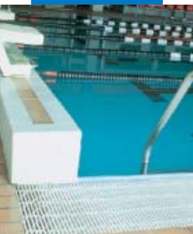
An example of an installation of mosaics with Keracrete + Keracrete Powder in a swimming pool
