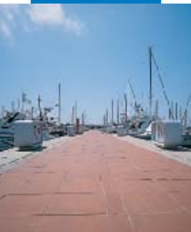
New harbor in Civitavecchia: outdoor installation of terracotta with Keracrete
