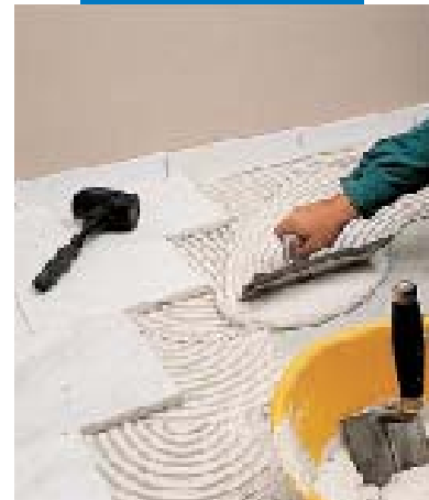
Laying white Carrara marble with Granirapid white
