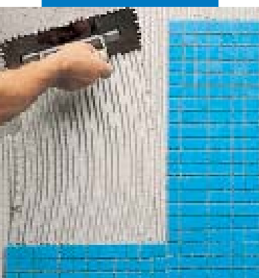
Laying vitreous mosaic with Granirapid white
