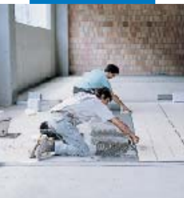
Laying porcelain tiles in a factory
