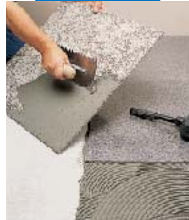
Laying synthetic flexible granite with Granirapid grey
