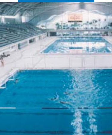
An example of an installation of mosaic and klinker in a swimming pool - Olympic Centre - Sydney (Australia)
